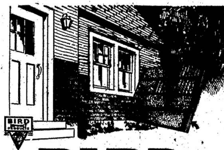
BIRD INSULATED BRIC SIDING
