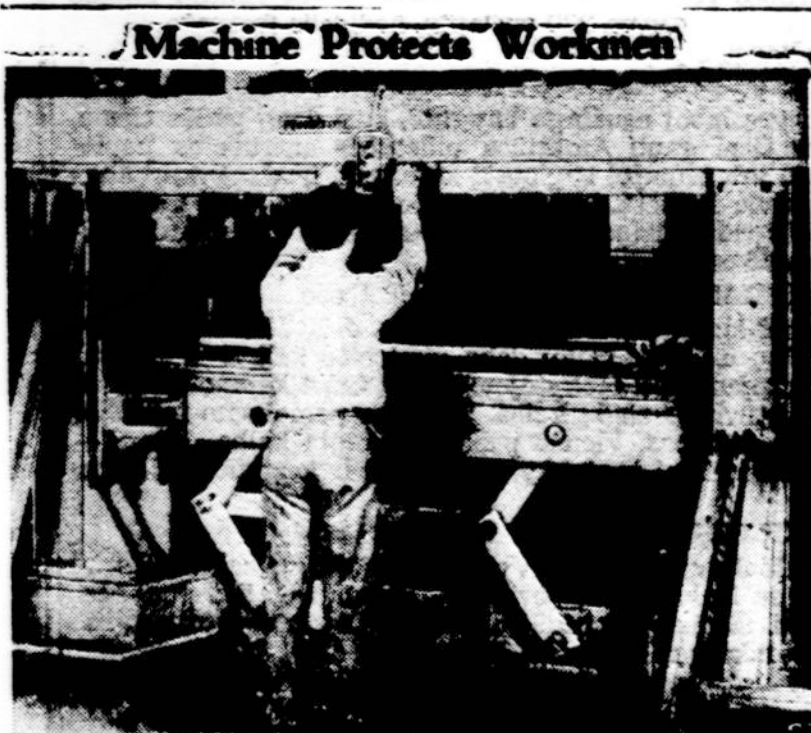
Safety is a feature of this new automatic welding machine, one of a battery recently installed by Fruehauf Trailer Company for multiple spot-welding of all-metal door frames. To start the machine, each operator must raise his hands and press two starting buttons simultaneously. This precaution guards against the possibility of either man having his hands in the machine when it starts operation.
