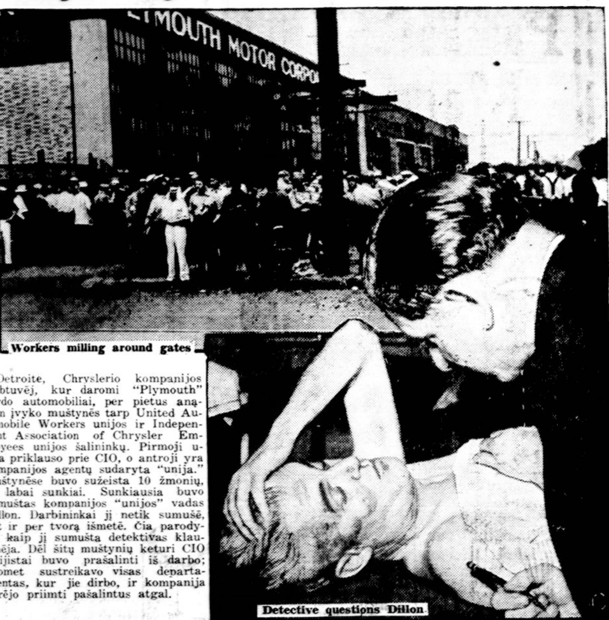
Workers milling around gates
