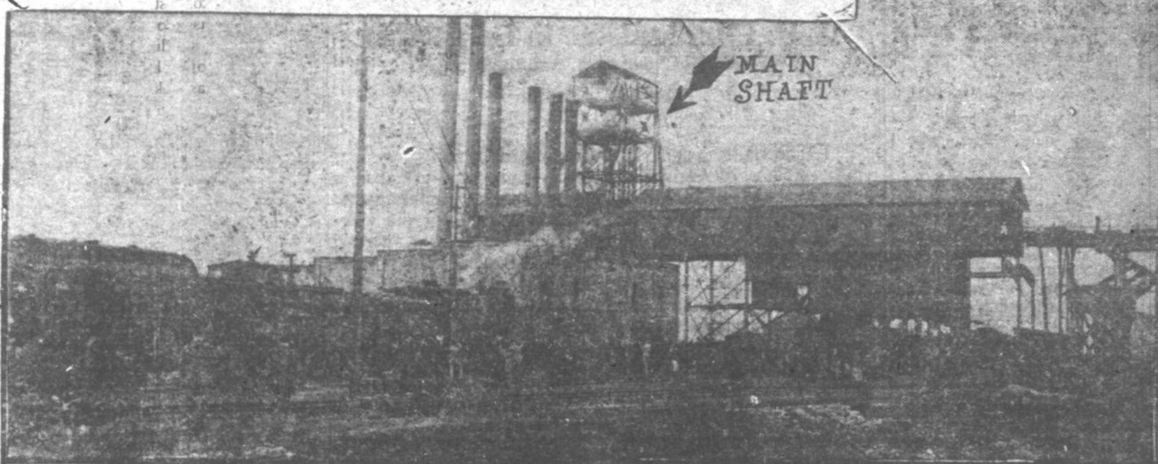
GENERAL VIEW OF SITE
