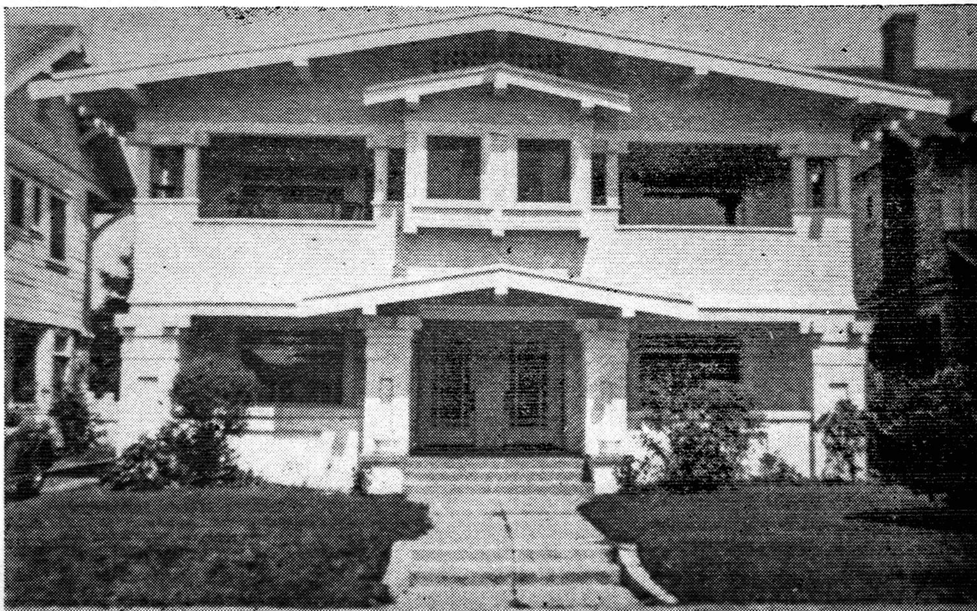
The Naginis residence at 1532 5th Ave., Los Angeles, California
