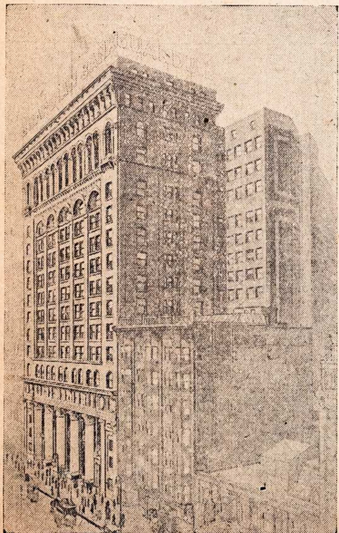
MAIN OFFICE—623 EUCLID AVENUE.
