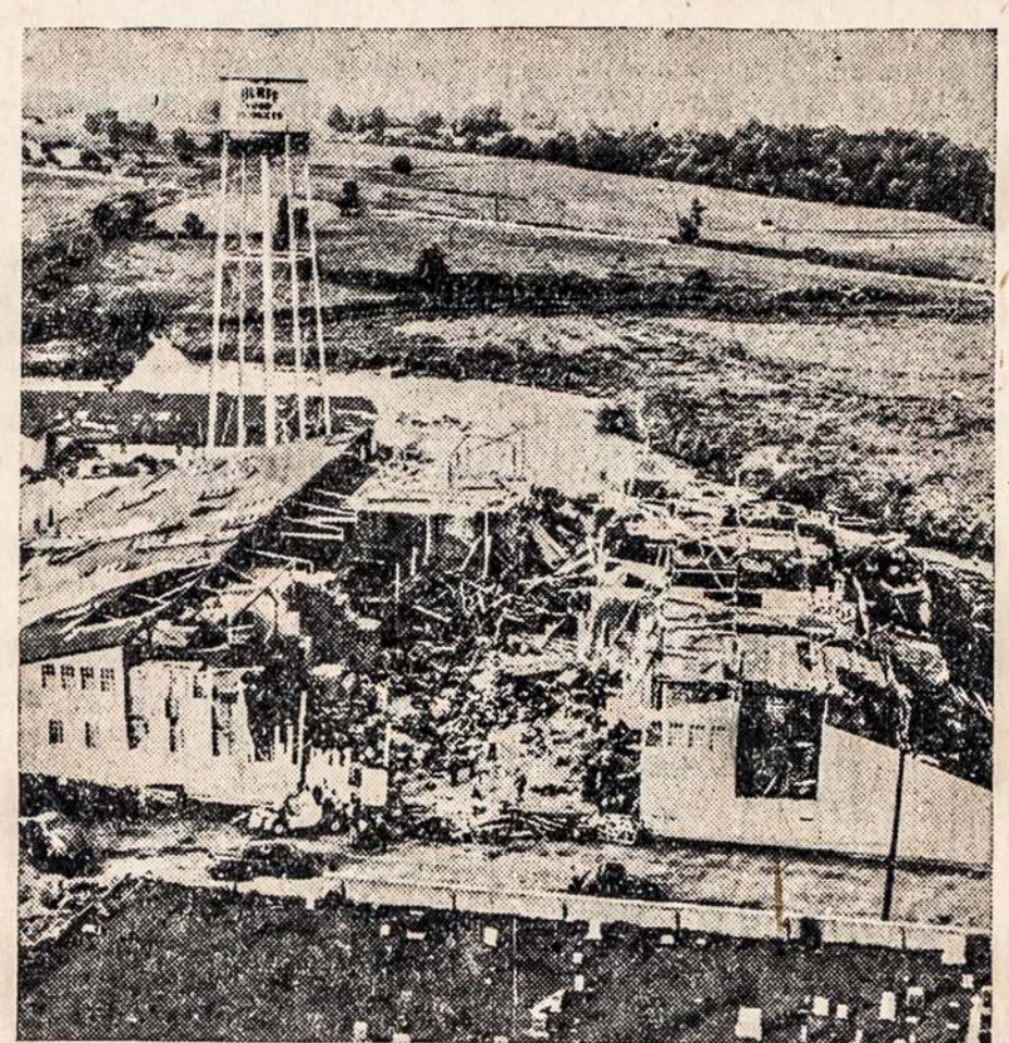
Shown here are the ruins of a canning factory at Swedesboro, N. J., after a tornado had ripped it to pieces. George Hemple, of Swedesboro, was crushed to death when a 150-foot steel stack at the cannery fell on and smashed the truck in which he was sitting. Eighty others were injured in the cannery. Other sections of Delaware and New Jersey suffered damage from the storm.
