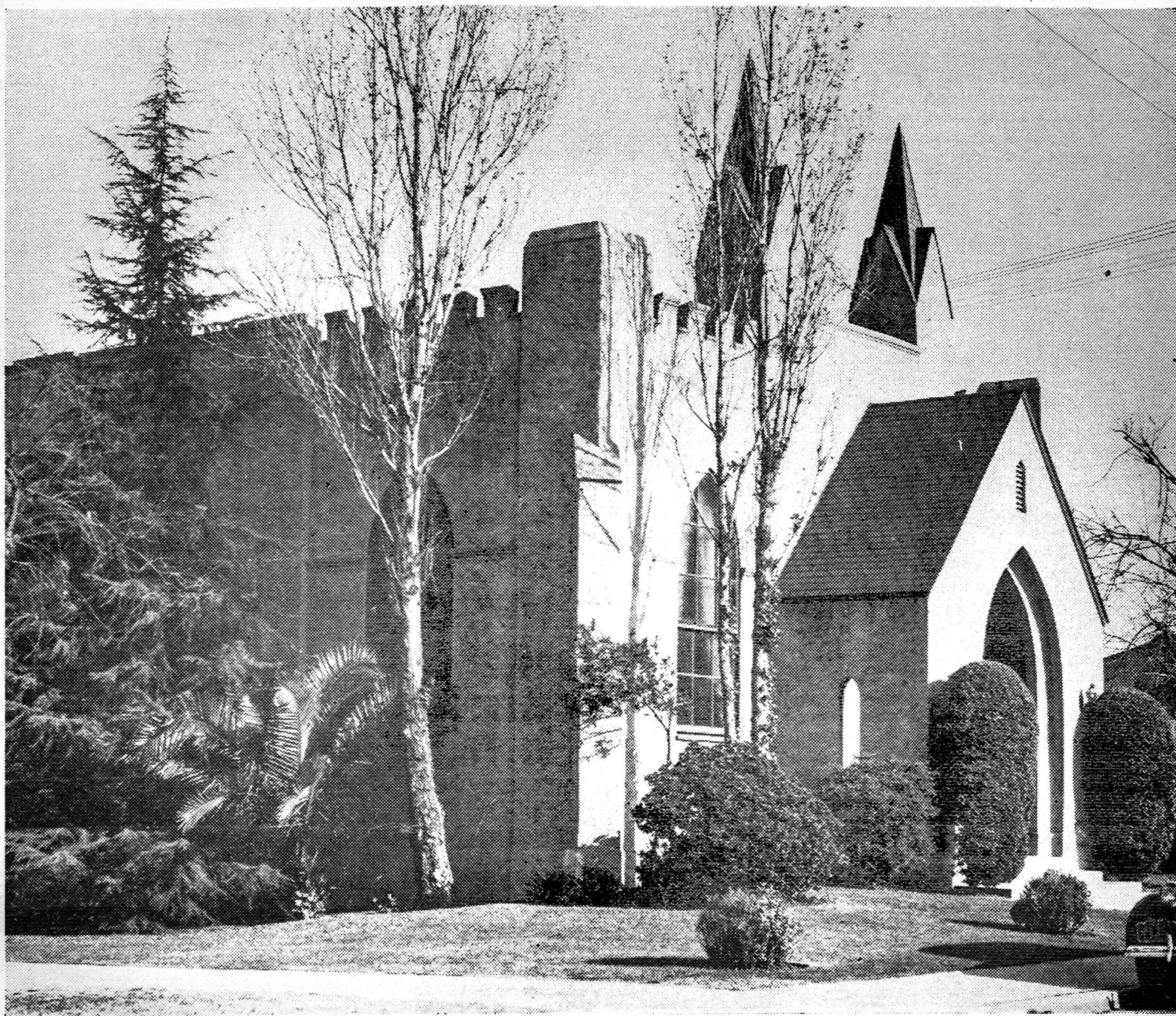
THE NEW ST. CASIMIR'S LITHUANIAN CHURCH IN SILVER LAKE DISTRICT, LOS ANGELES, CALIFORNIA
