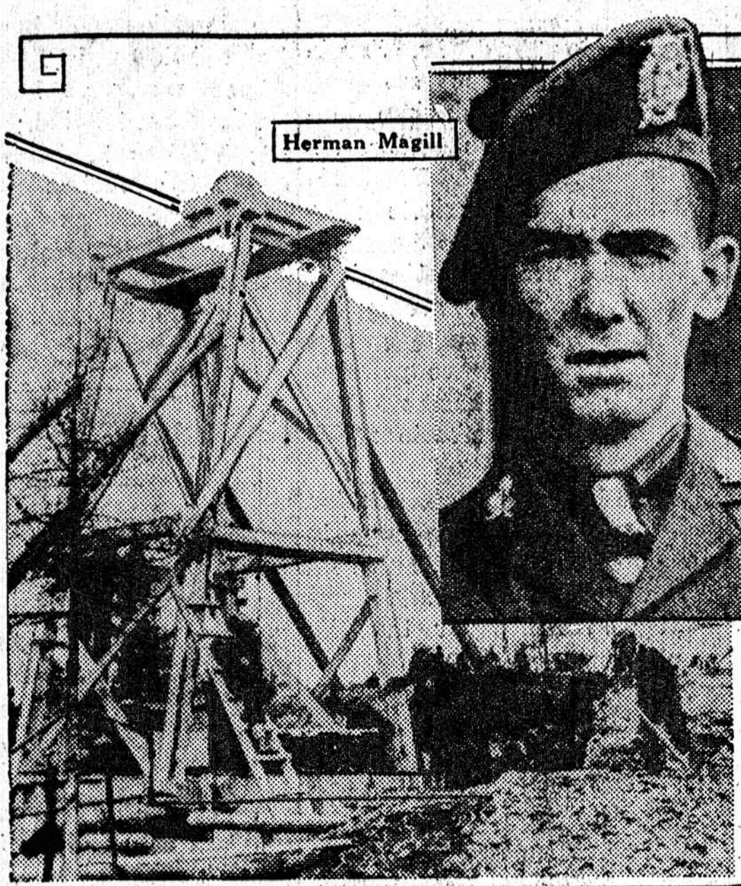
Derrick above emergency shaft
