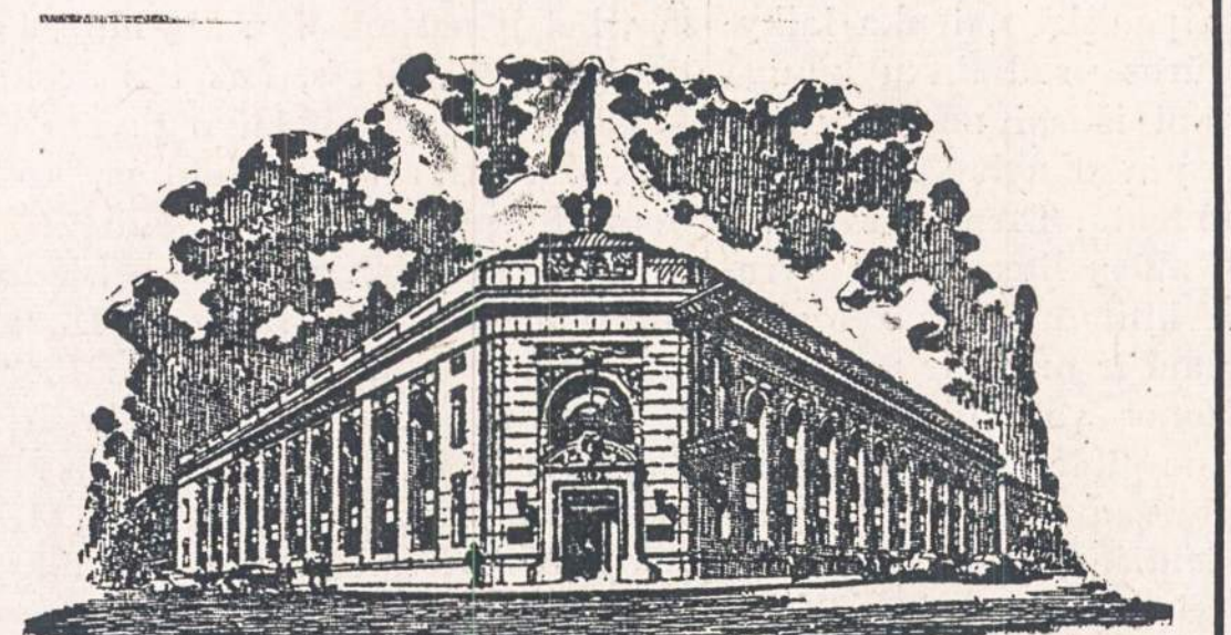
Standard Federal Building.
