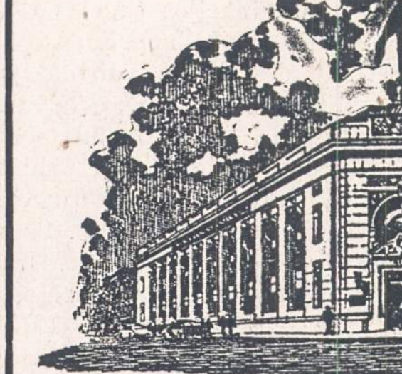
Standard Federal Building.
