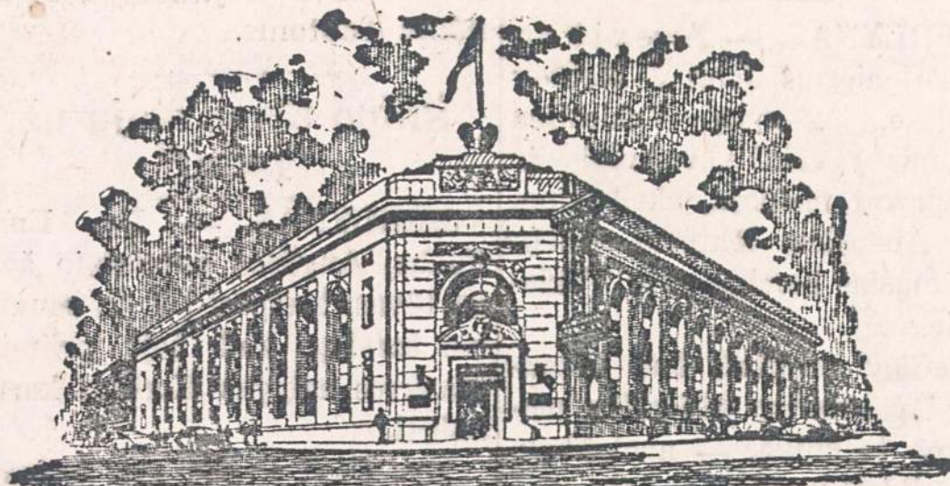
Standard Federal Building.
