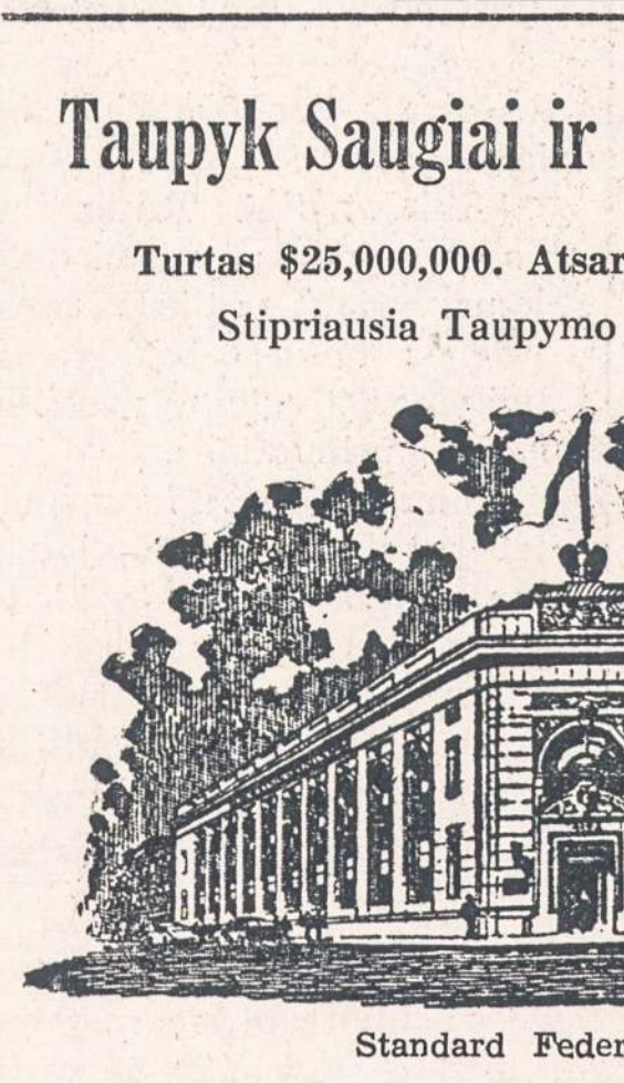
Standard Federal Building.
