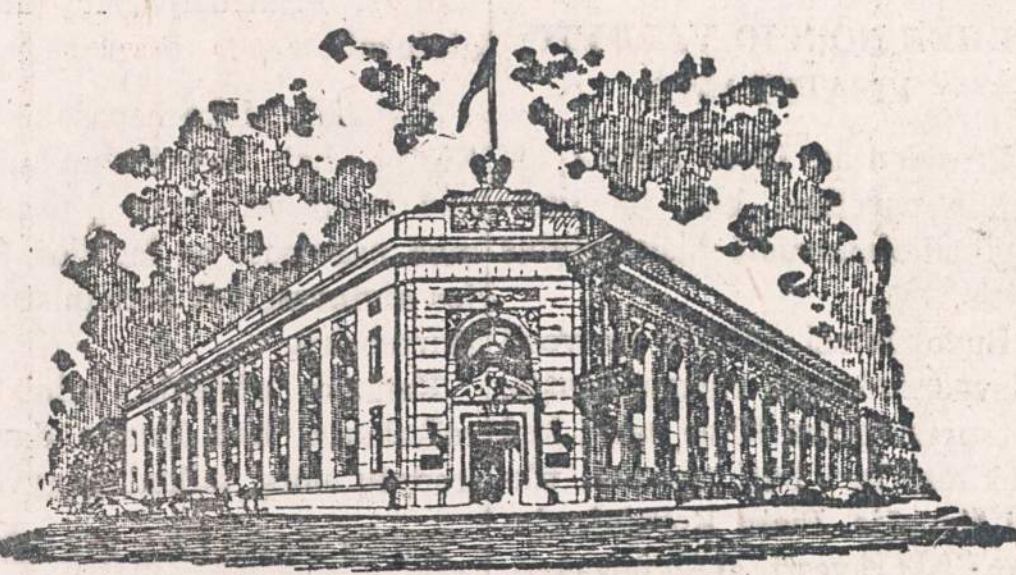
Standard Federal Building.
