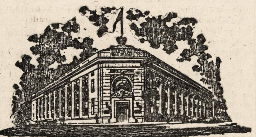
Standard Federal Building.
