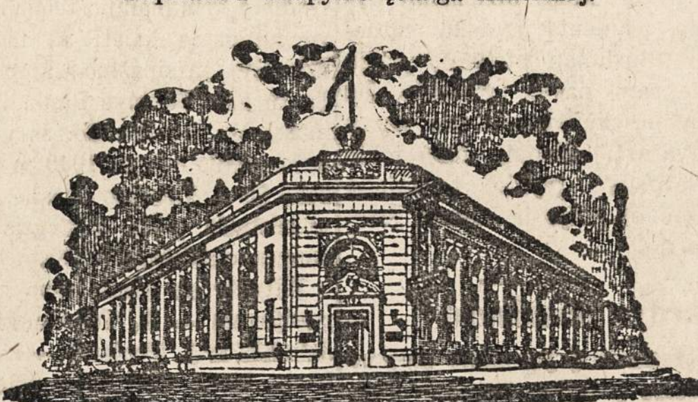
Standard Federal Building.
