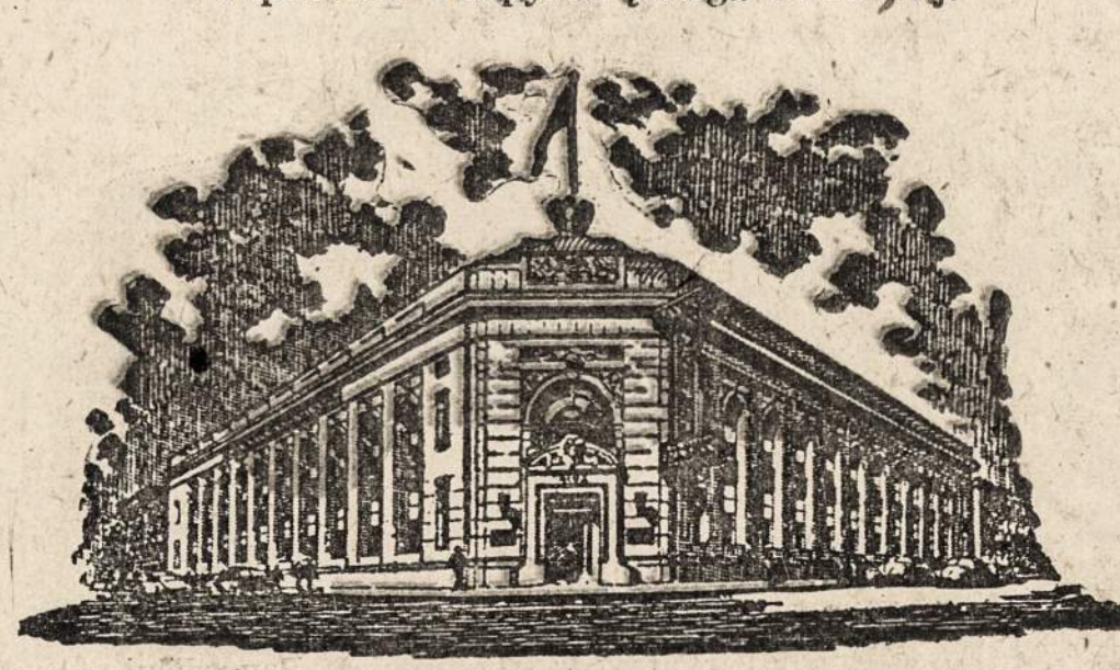
Standard Federal Building.
