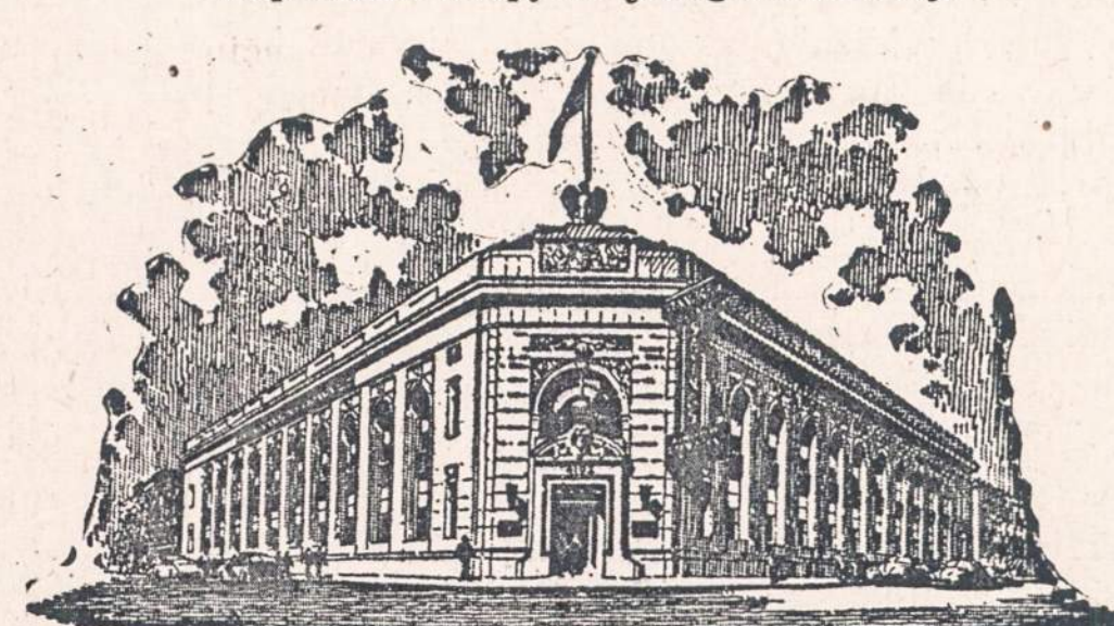
Standard Federal Building.
