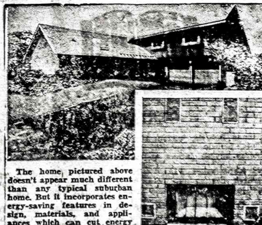
The home, pictured above doesn't appear much different than any typical suburban home. But it incorporates energy-saving features in design, materials, and appliances which can cut energy needs by up to 50 percent. It has two heat-circulating Heatilator fireplaces (right), designed to draw room air in through the lower vents, warm it and then re-direct the heated air back into the room.
