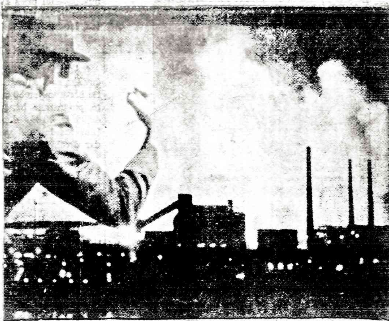
Pieno liejyklos South Works fabrikai
