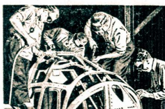
At Willow Run the top section of the bomber's enclosure, formerly made in 13 hand-formed pieces — is now made in only 3 parts — saving 30 hours in the construction time of each bomber.
